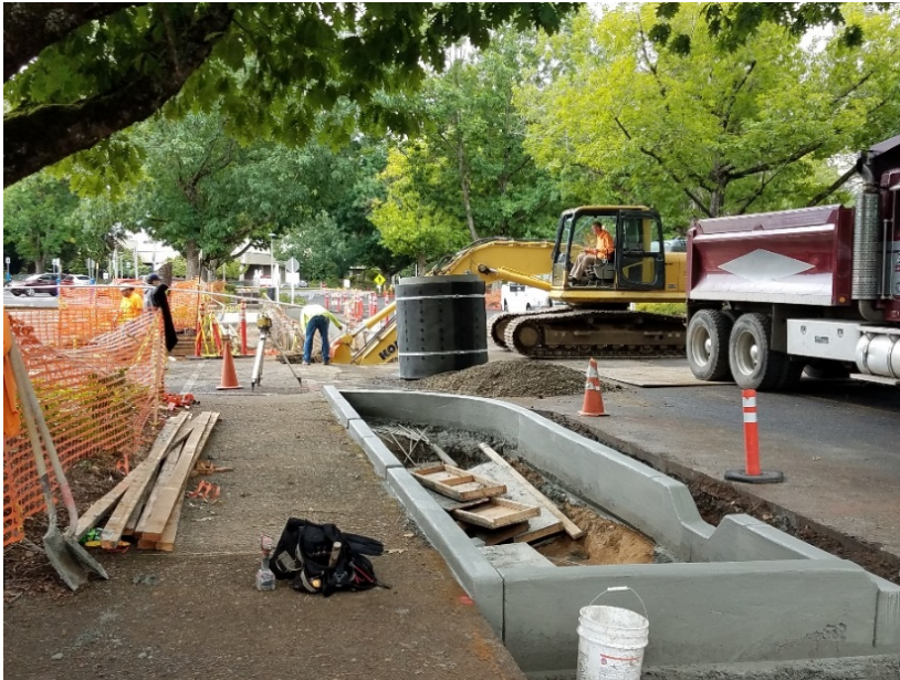
Figure 5: Installation of drywells at MHCC
