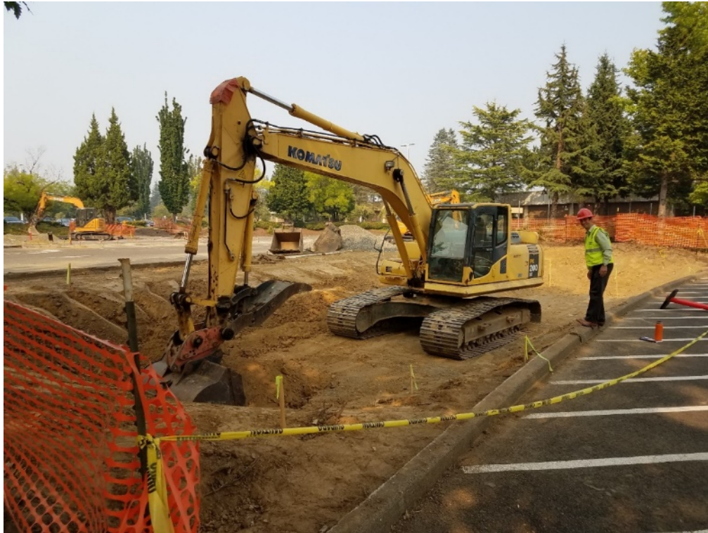
Figure 4: MHCC Large raingarden before and after construction
